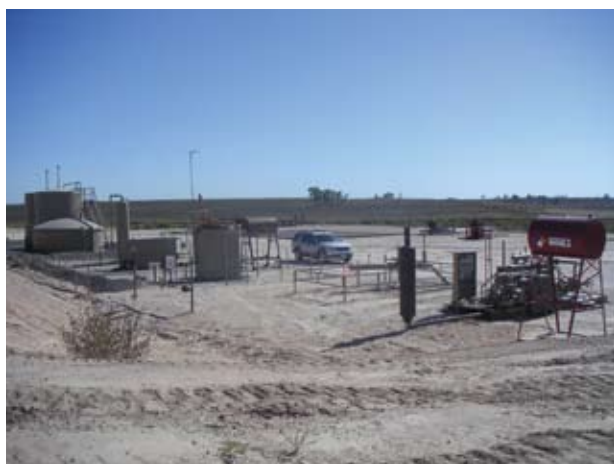
Kelln Trust 5-1 Site Facilities.
